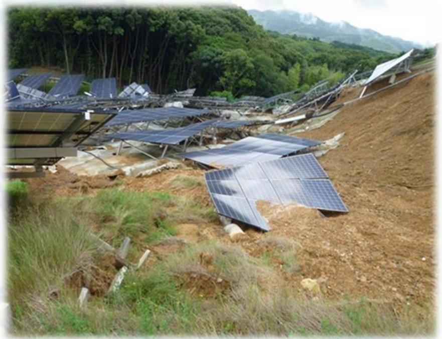
Landslide damage due to heavy rain
